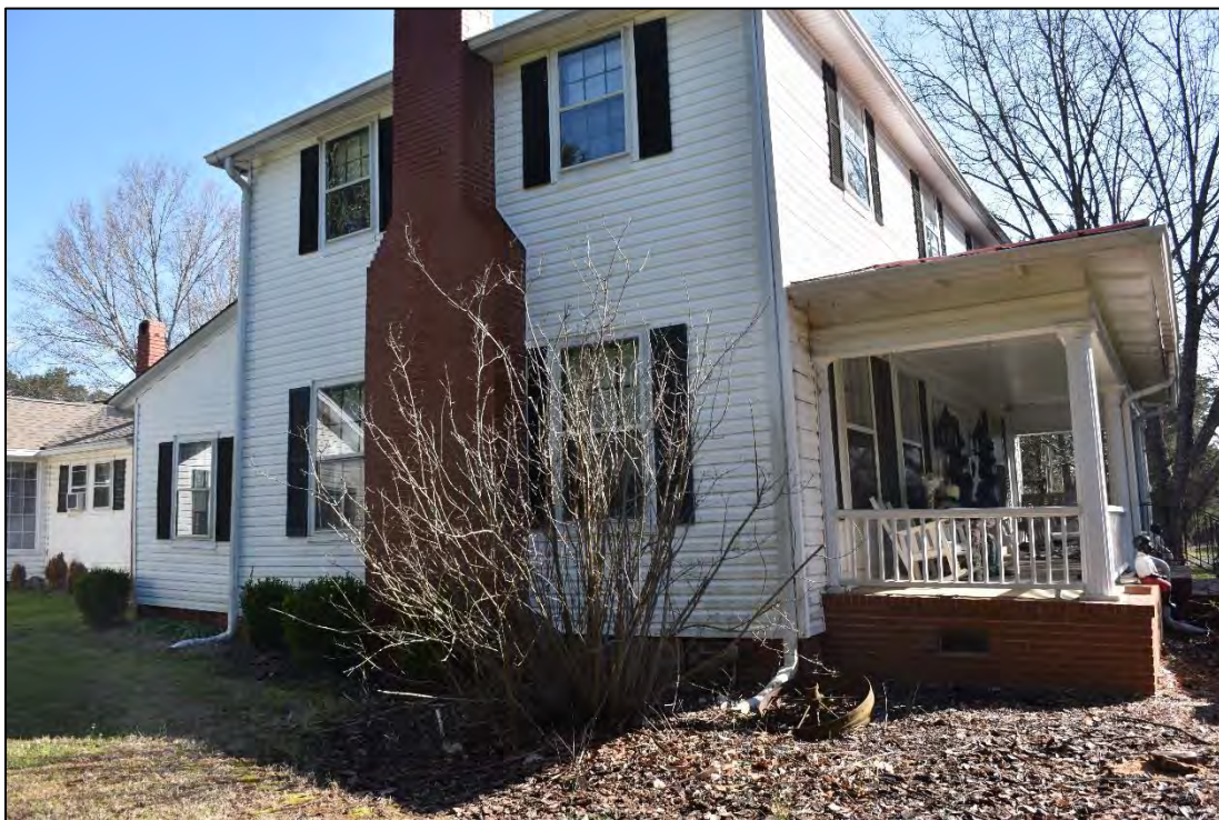
Figure 2.6. Blackwelder-Litaker House, facing northeast.
