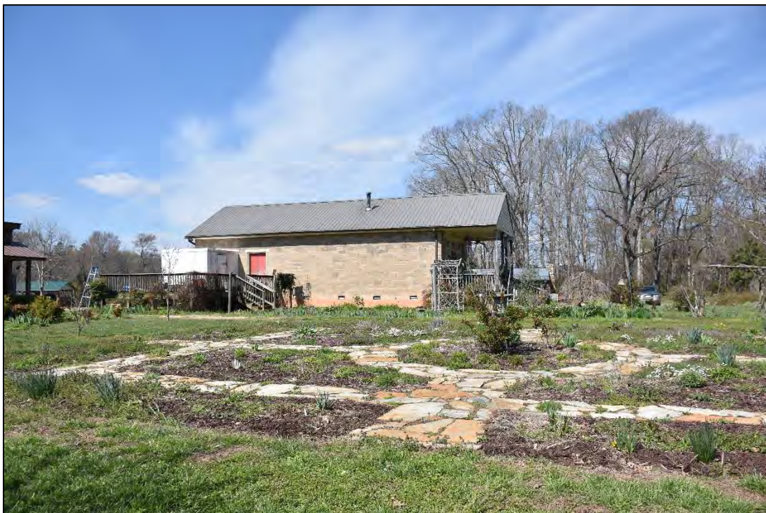
Figure 2.74. Bradford Store, facing west.
