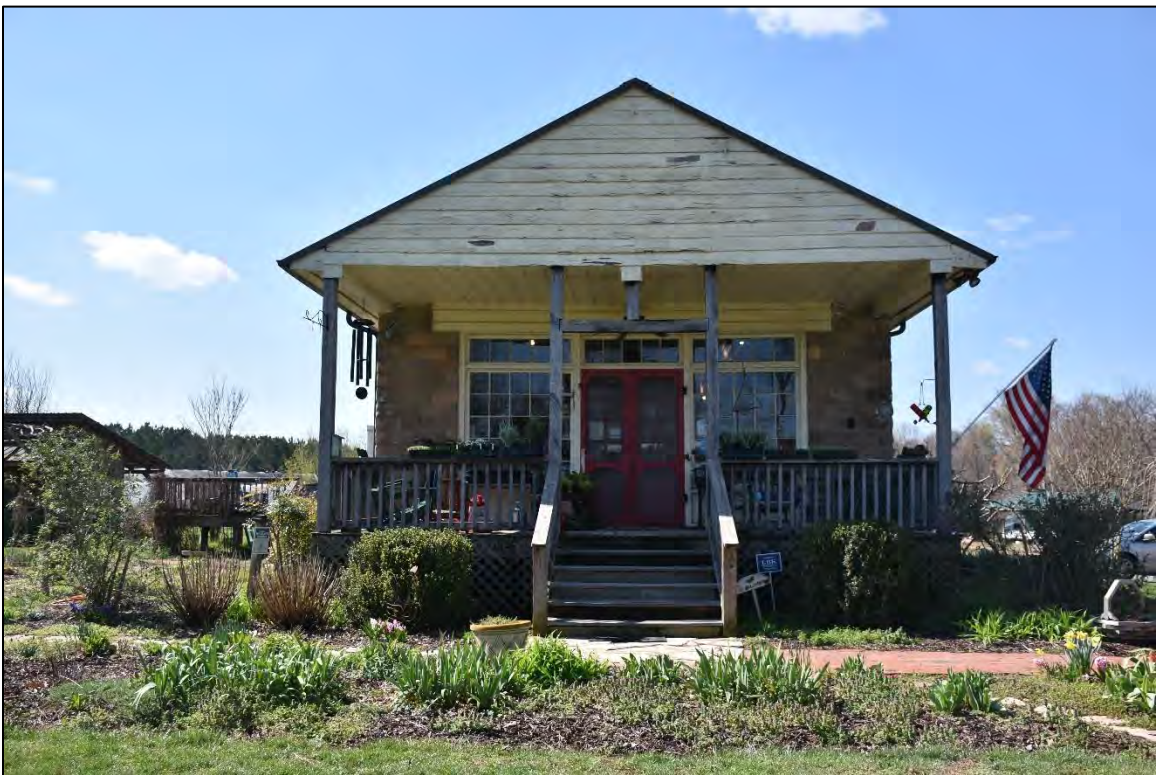
Figure 2.72. Bradford Store, facing south.
