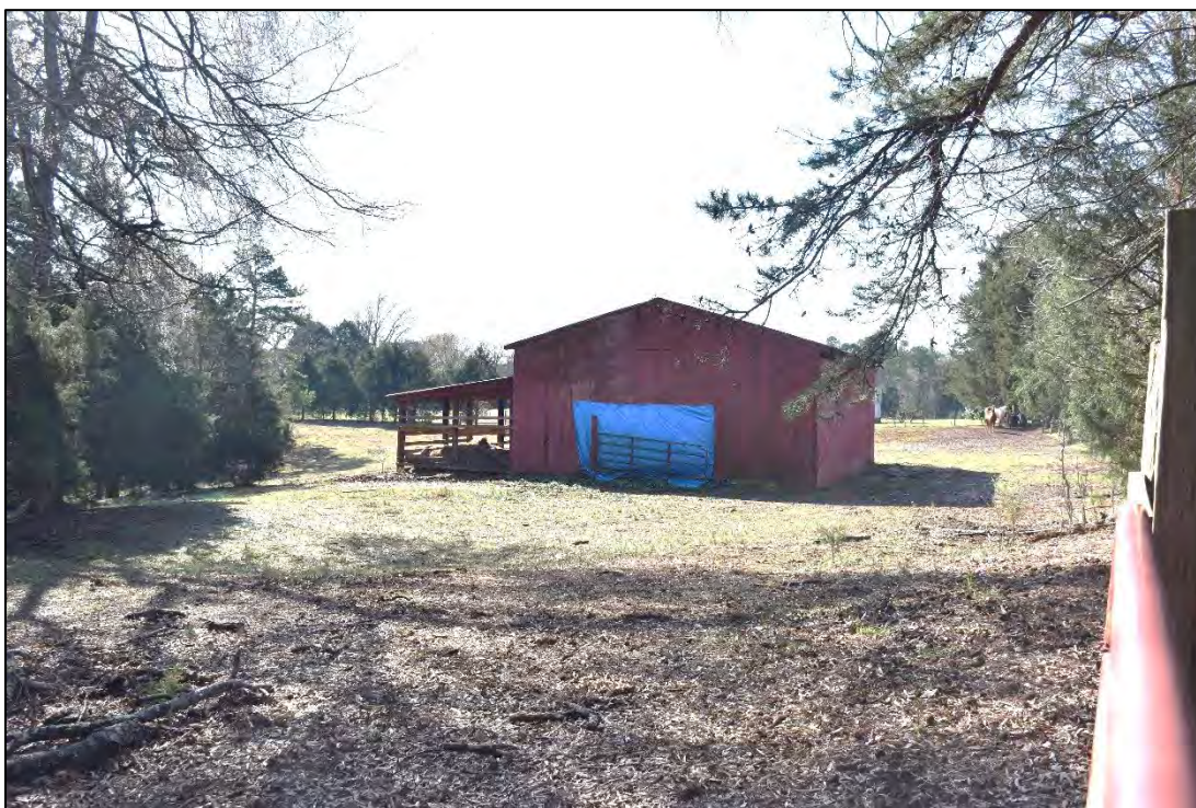
Figure 2.27. Barn, circa-1920, facing southeast.
