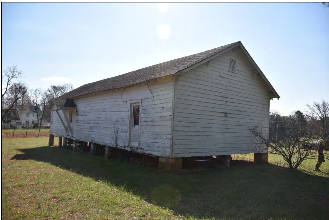
Figure 2.16. Current storage building, circa-1920, rear elevation facing southeast.
