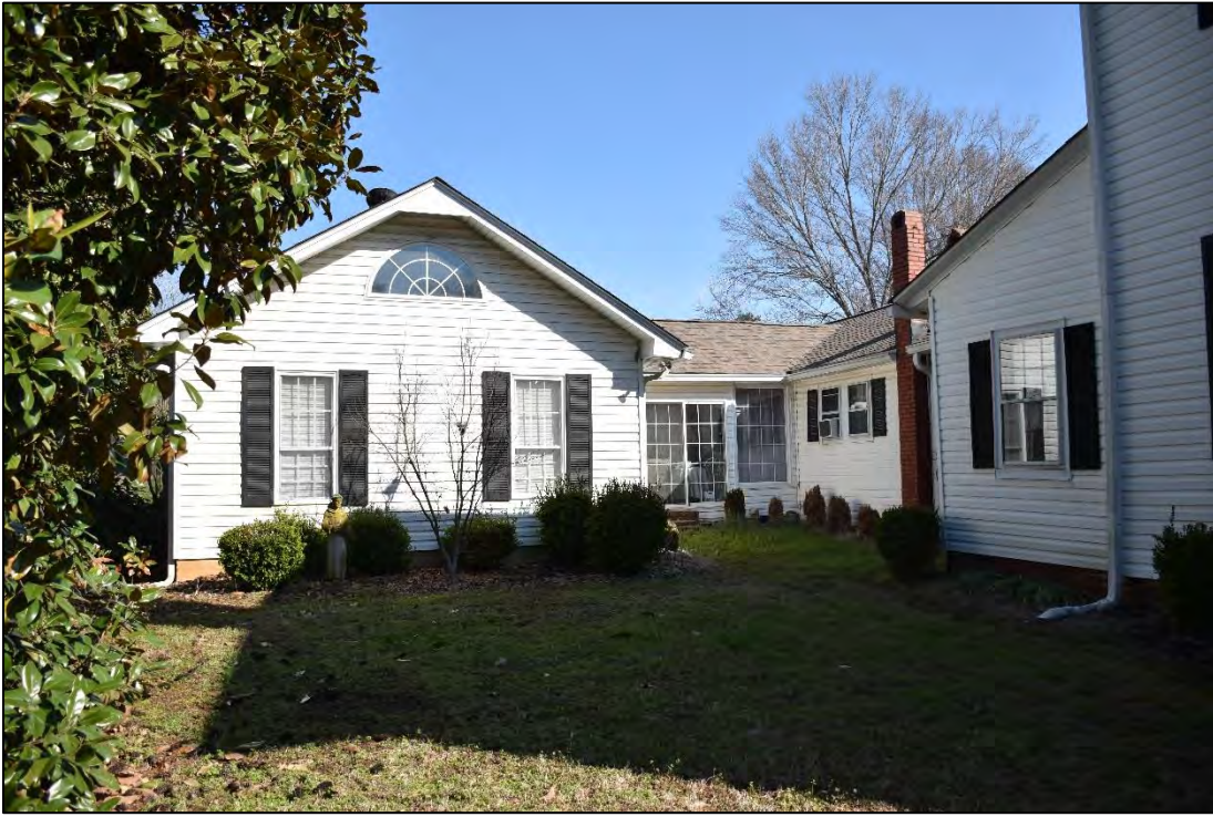
Figure 2.10. Blackwelder-Litaker House, facing northeast.
