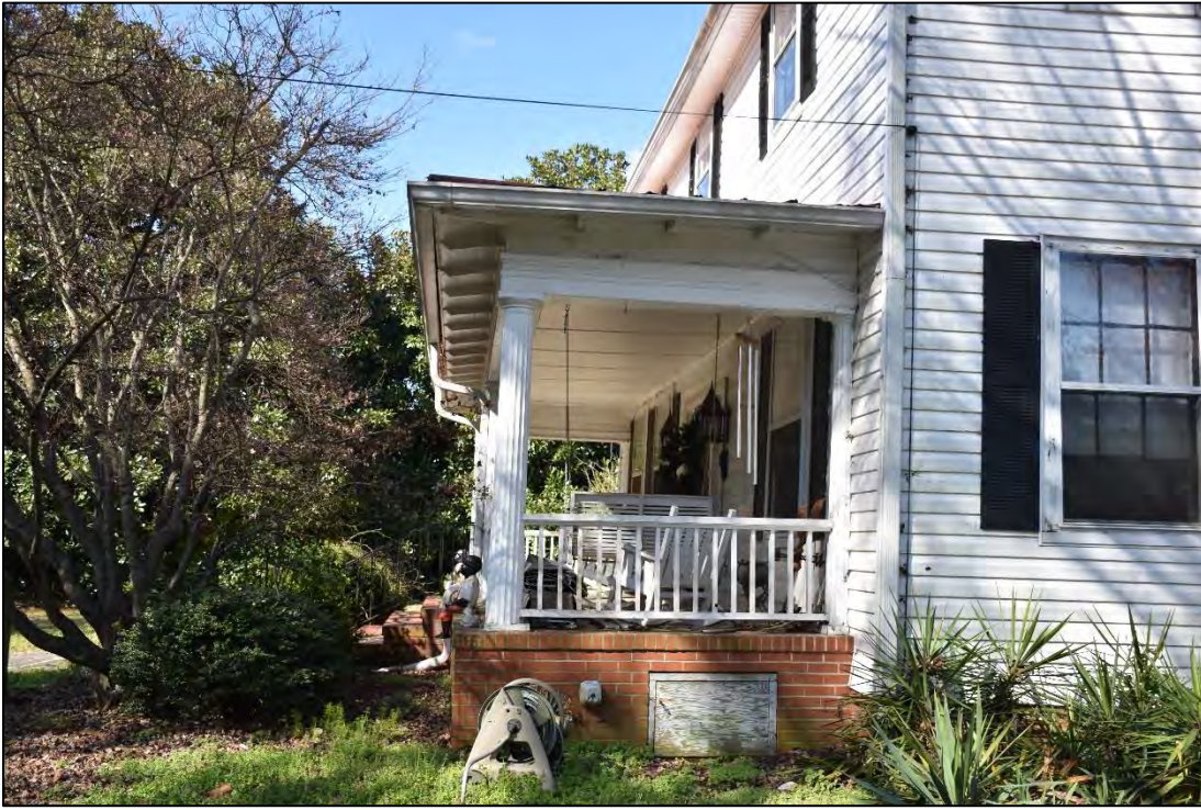
Figure 2.3. Blackwelder-Litaker House, porch detail, facing west.
