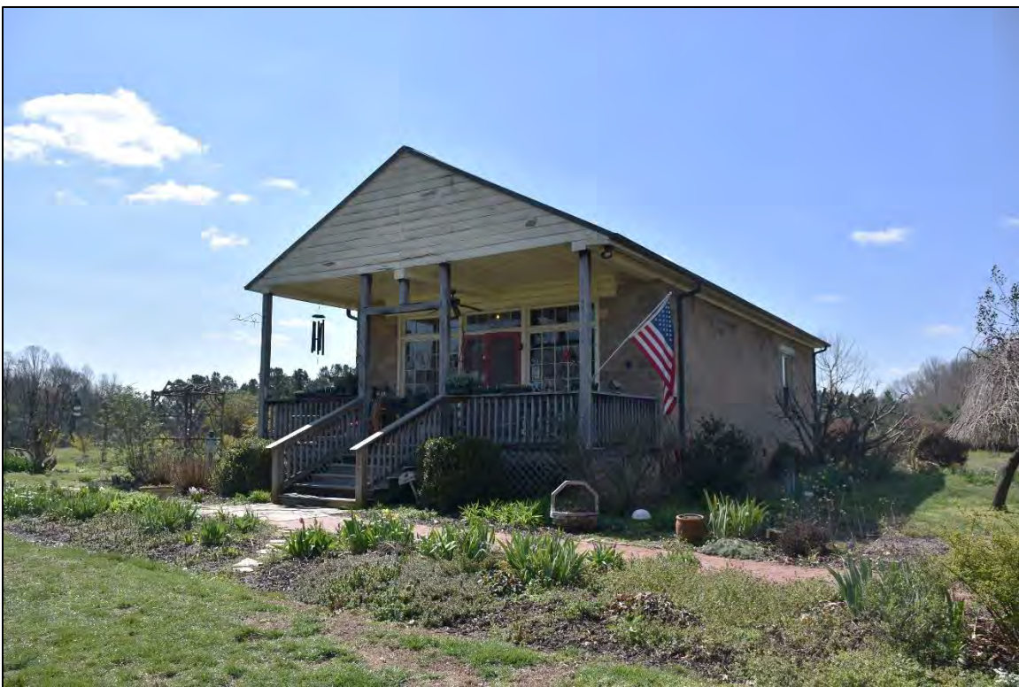
Figure 2.71. Bradford Store (MK2811), facing southeast.
