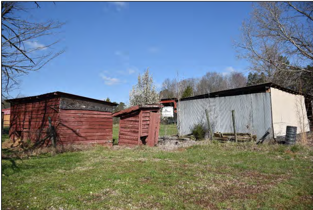
Figure 2.29. Storage buildings and outhouse, circa-1900 through 1960s, facing northwest.
