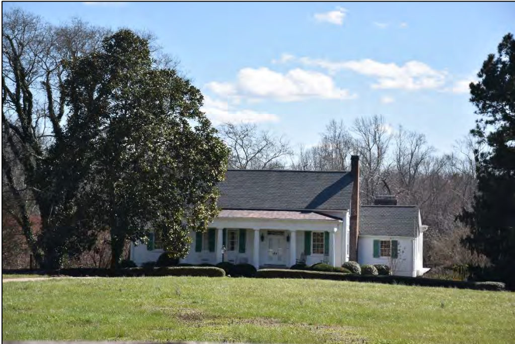
Figure 2.41. Mill Hill (CA0003), facing south.
