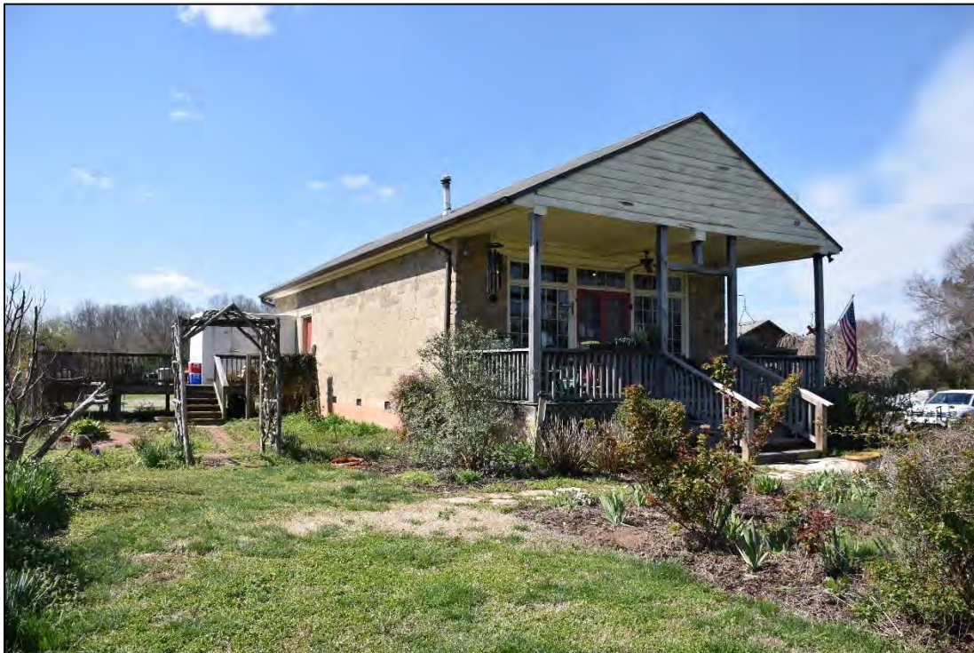
Figure 2.73. Bradford Store, facing southwest.
