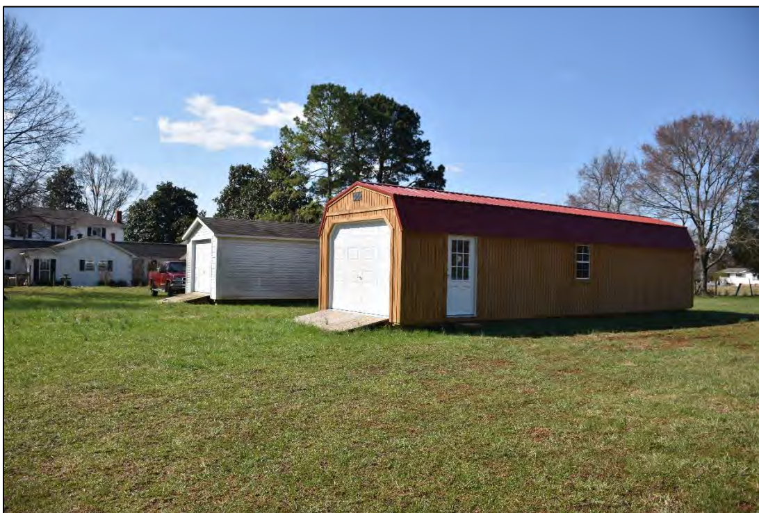
Figure 2.34. Modern storage buildings, facing southwest.
