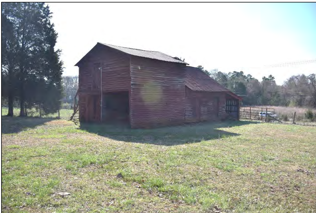
Figure 2.11. Barn, circa-1900, facing southeast.
