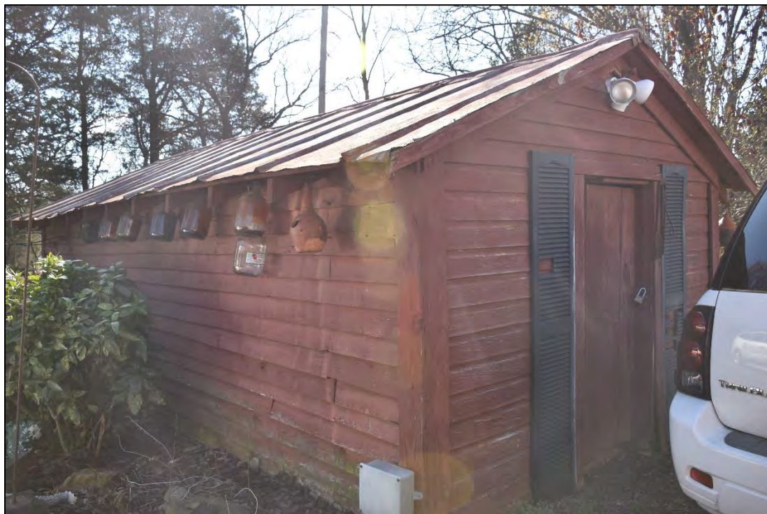
Figure 2.19. Shed, circa-1930, facing east.
