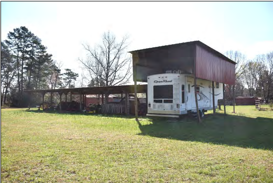
Figure 2.33. Open storage, circa-1970s, facing south.
