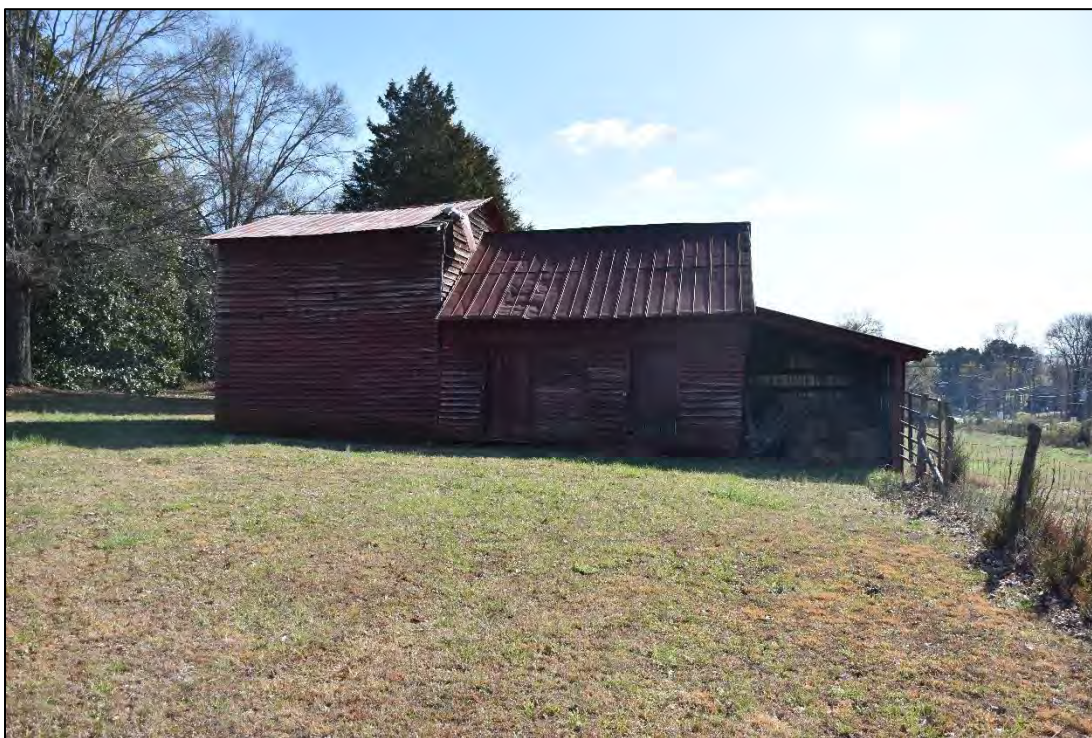
Figure 2.12. Barn, circa-1900, facing east.
