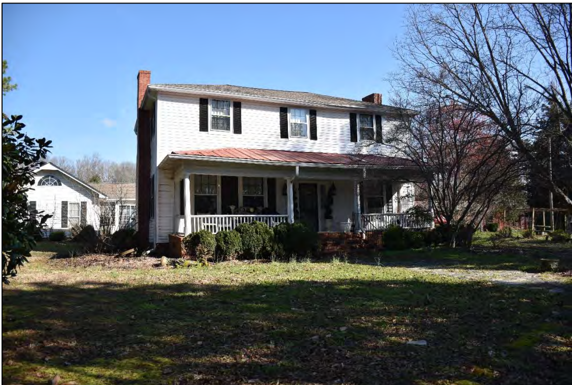
Figure 2.1. View of the Blackwelder-Litaker House, facing north.
